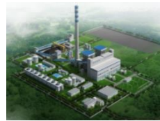
2x300 MW Peranap Power Plant
