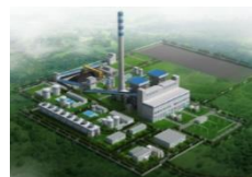
2x350 MW Kuala Tanjung Power Plant
