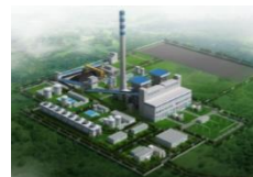
2x300 MW Sumsel 6 Power Plant
