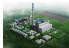
2x40 MW Halmahera Timur Power Plant
